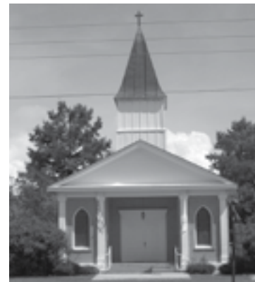
ST. FRANCIS OF ASSISI MISSION CHURCH, WATERPROOF, LA
